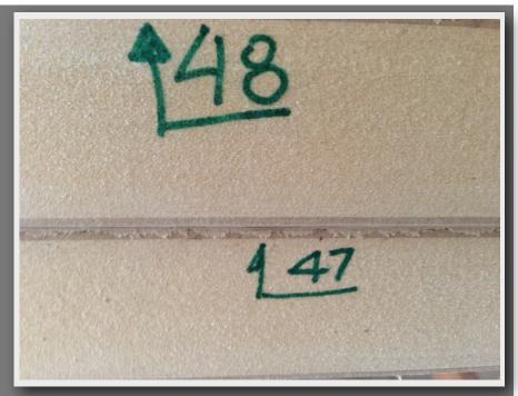
Mark the bottom edge of the door with sequence numbers so as to insure correct matching on the job site.
