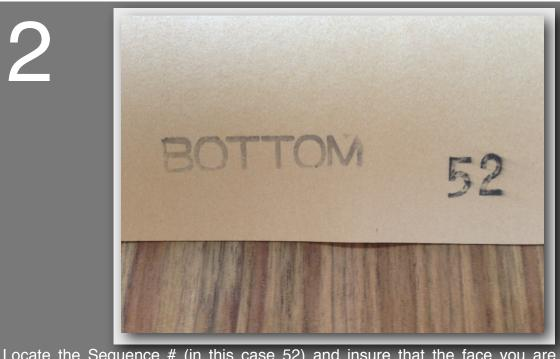
Locate the Sequence # (in this case 52) and insure that the face you are about to bond is the correct face for the elevation you are working on. Be certain that the sheet is oriented correctly.
